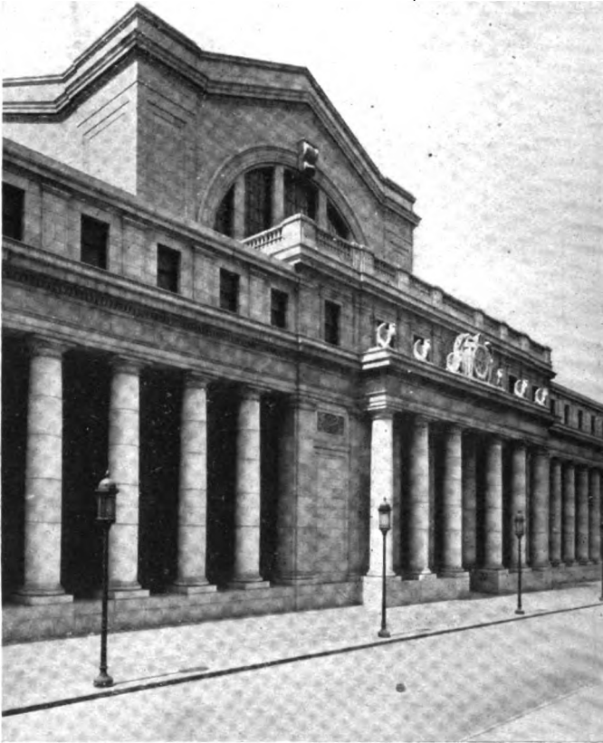
Detail of Thirty-third Street Entrance to Main Waiting-room
